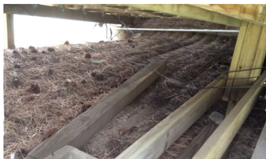
Open foundation with combustible debris
