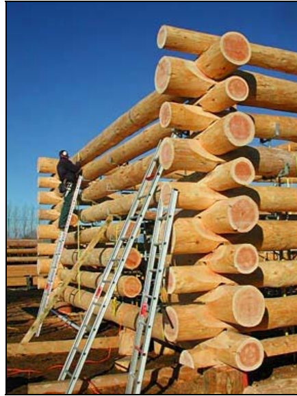
Figure 32. Log Shell Under Construction Using “Accelerated” Log Building Method.
