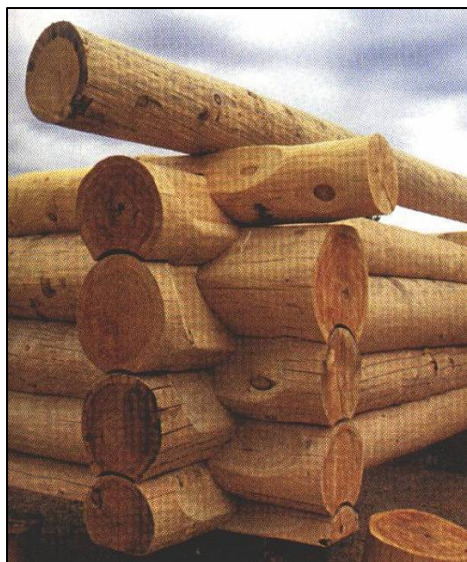
Figure 31. Traditional Method of Constructing Log Structures Fitting One Log at a Time.
