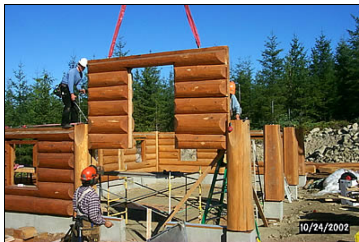
Figure 33. Home Being Built Using “Piece-on-Piece” Building Method
