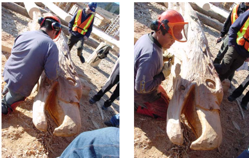
Figure 30. Worker Crafting an Architectural Feature for a Log Home
