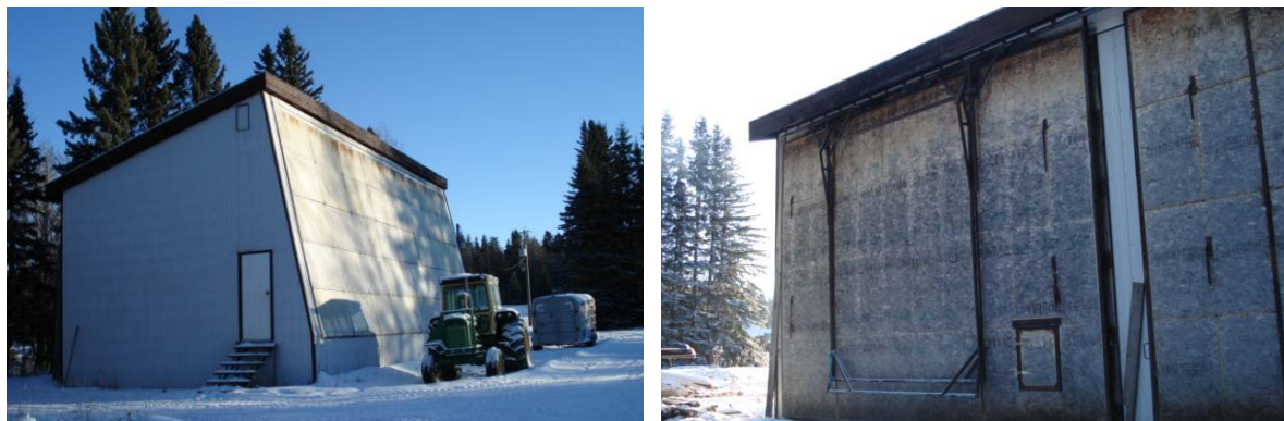
Figure 6. In-house Build Solar Kiln With Drying Capacity of 10,000 per charge
