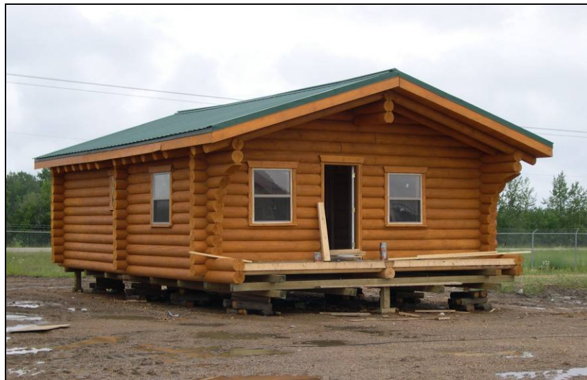
Figure 38. Portable Machine Profiled Log Home Built On Pressure Treated Skids
