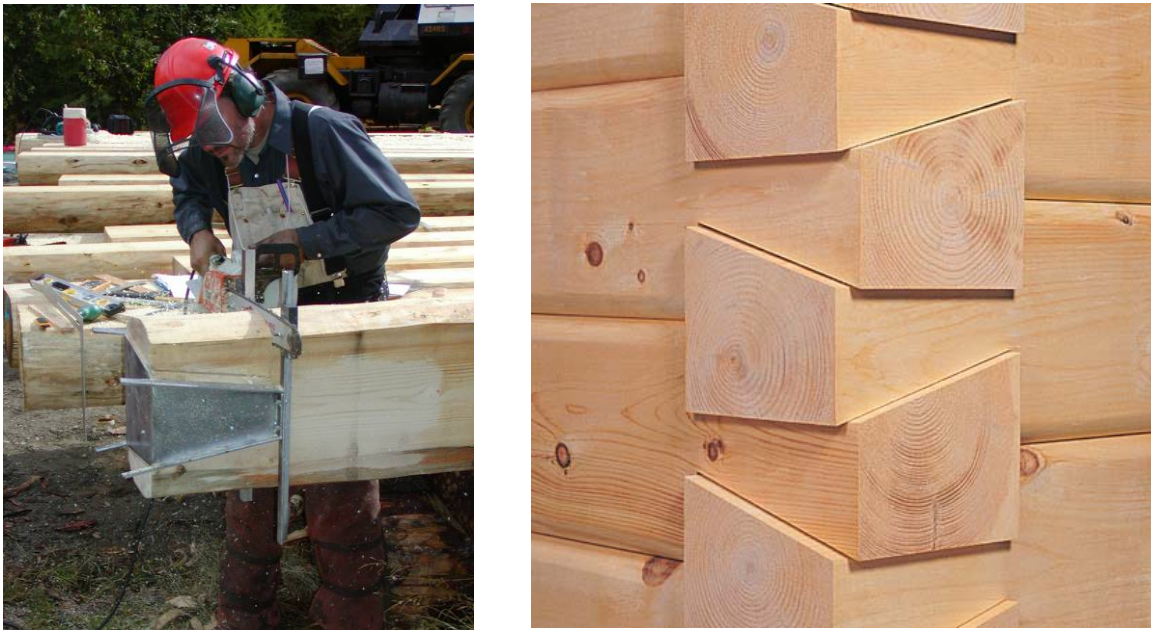
Figure 35. Cutting of Dovetail Corner Joint Using Jigs (l), Machine Cut Dovetail Joint (R)
