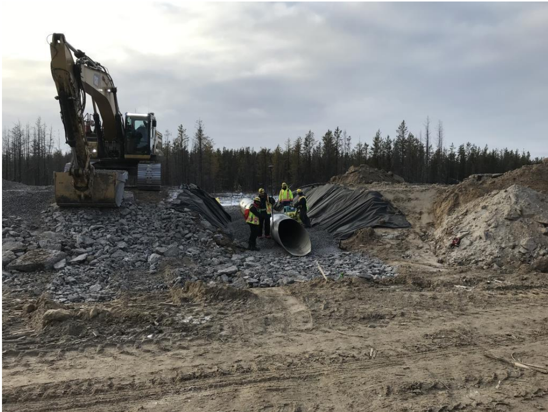
Photo 4. Culvert Installation at Station 7+850 on November 8 th , 2019.
