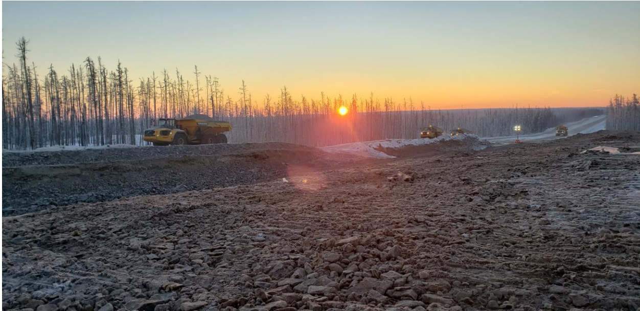
Photo 3. Haul trucks moving embanking materials for the placement.
