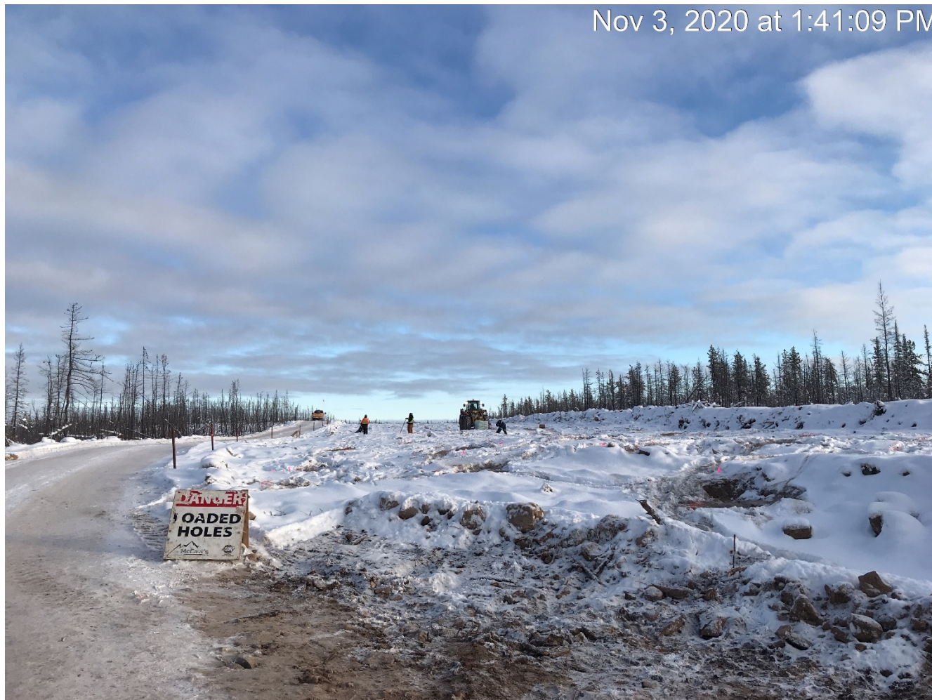
Photo 10. Looking south at the loading of holes for a blast at Station 94+690
