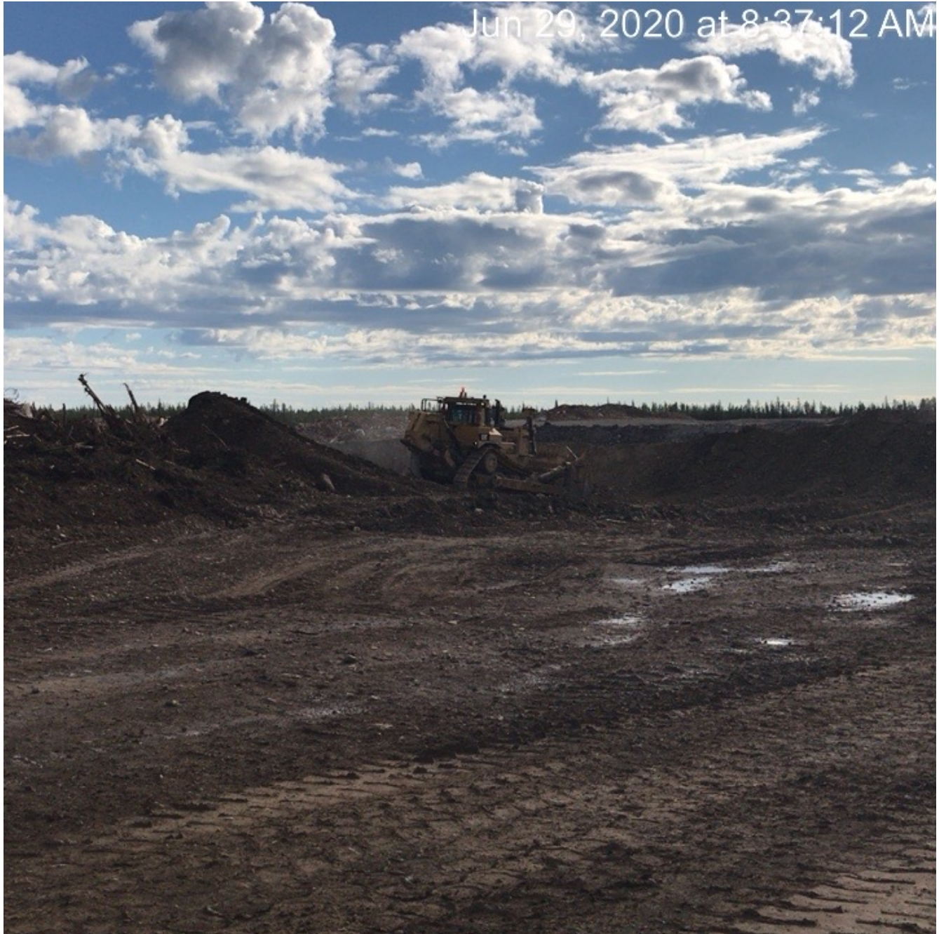
Photo 8. Looking northeast at the preparation of material at Pit 48
