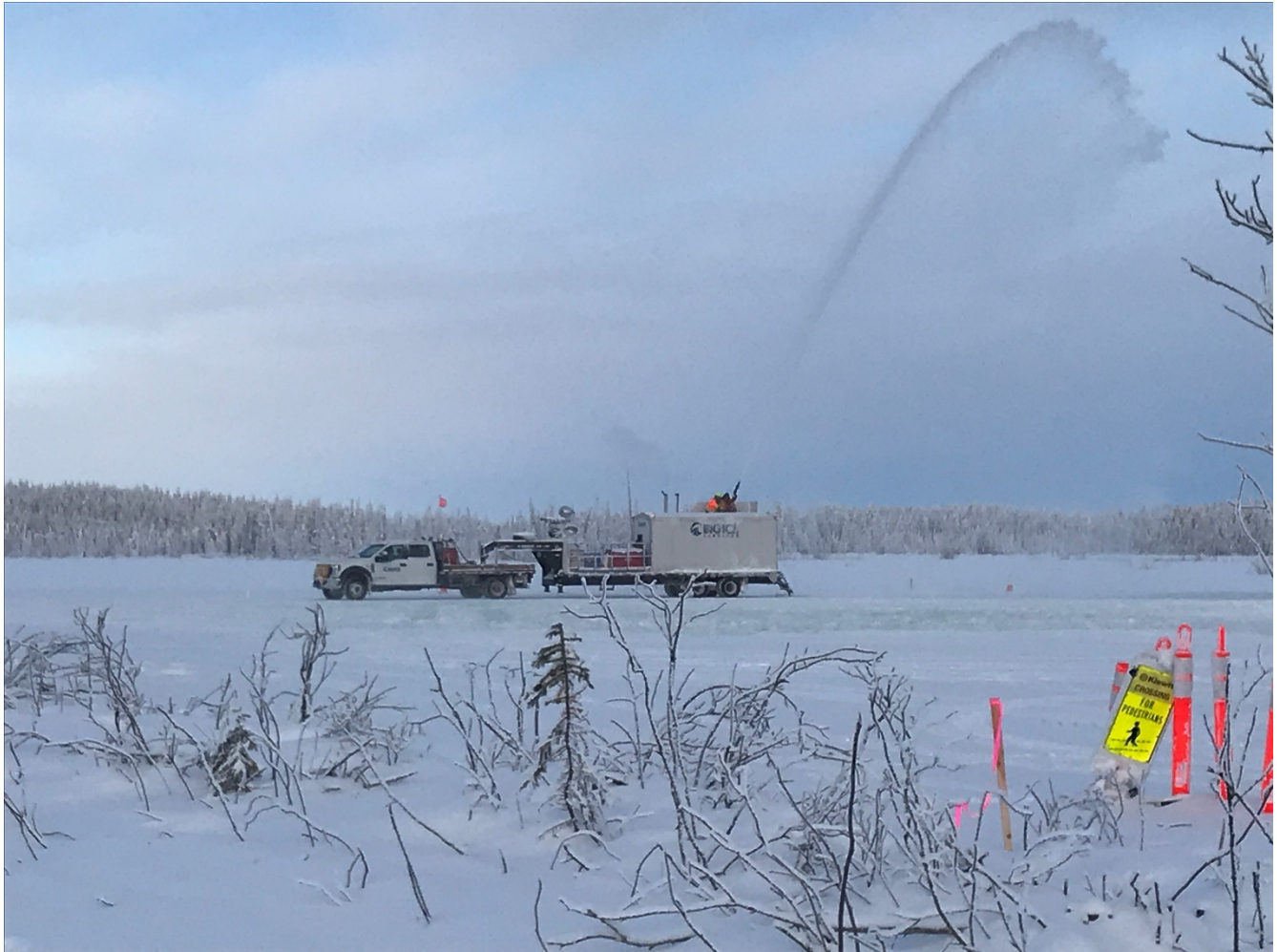
Photo 11. Big Ice applying water onto the ice crossing at the LaMartre River
