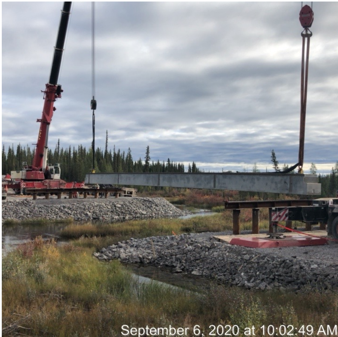
Photo 14. Looking east at girder placement at the Duport River structure.
