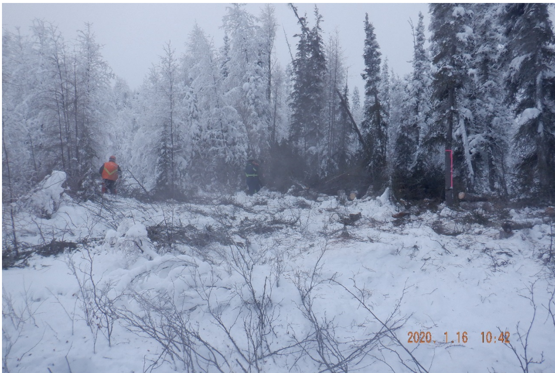
Photo 6. Looking west at hand cutting activities at James River Crossing
