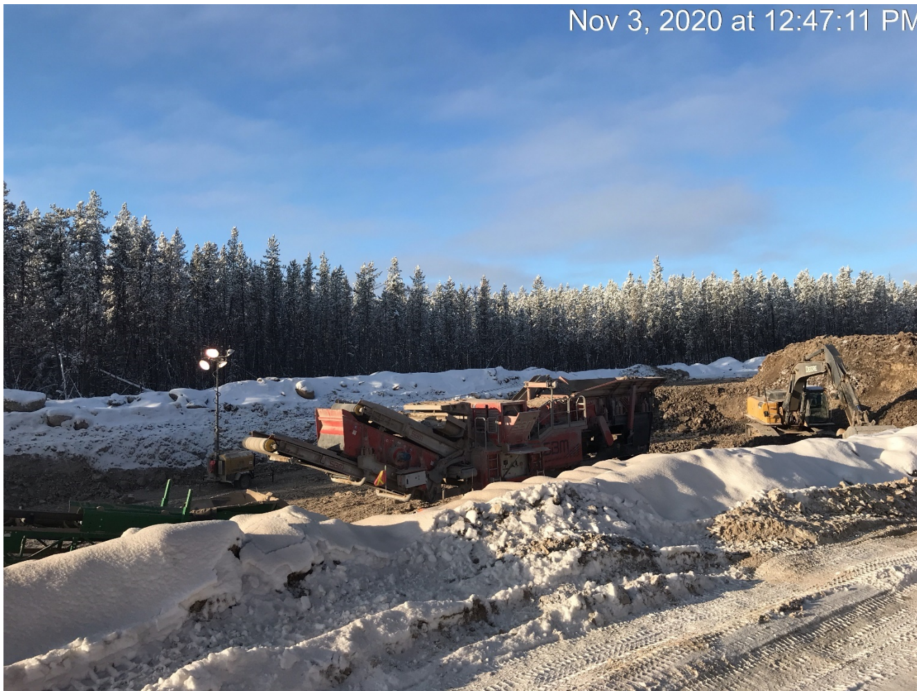
Photo 17. Looking north west at crusher operating in road cut at ~ Station 59+000.
