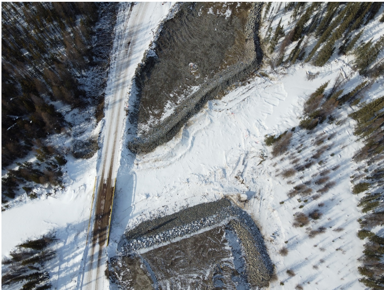
Photo 12. Overhead drone image showing the temporary crossing at the James River
