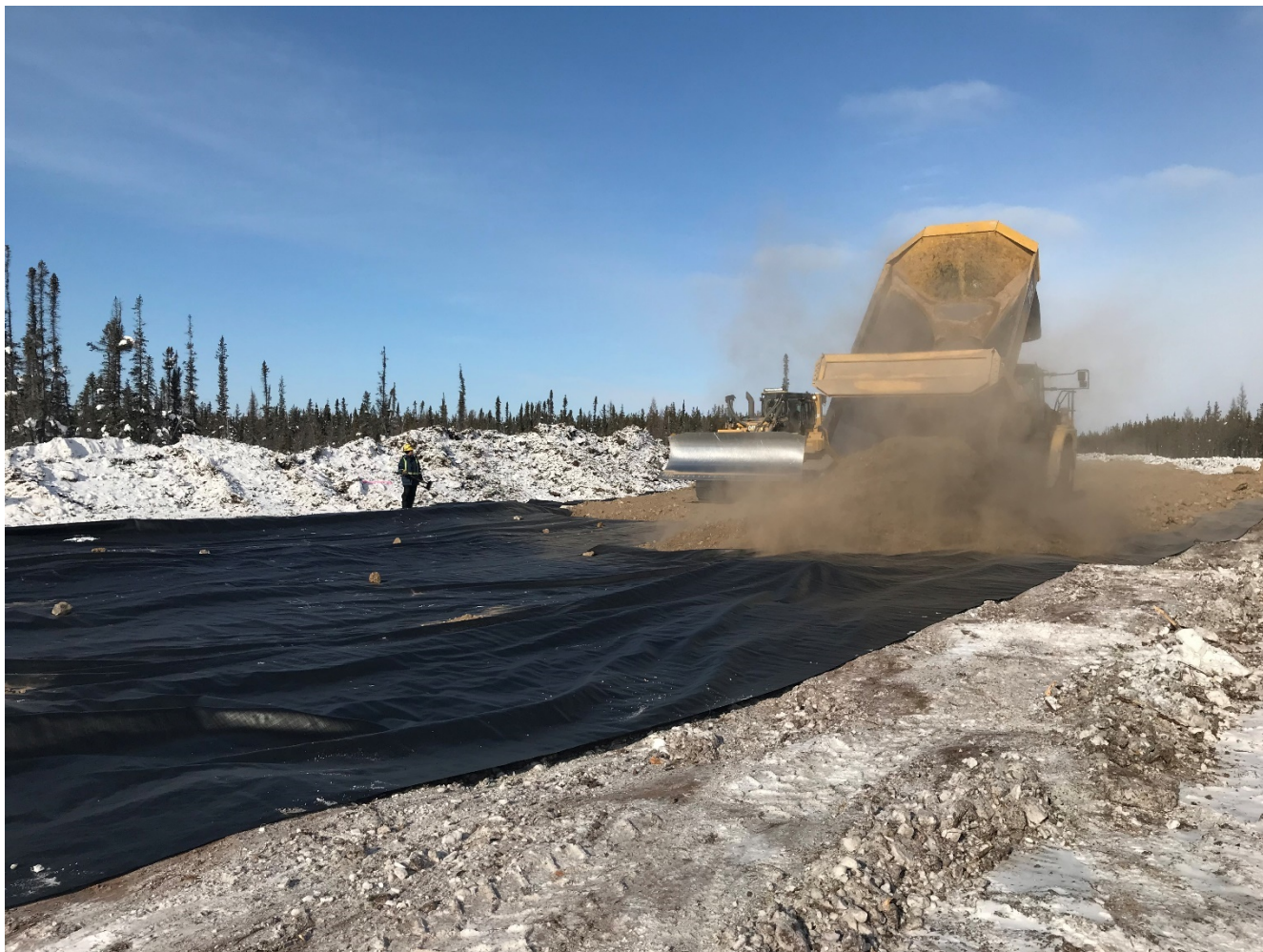
Photo 9. Embanking material being placed on geotextile at ~ Station 50+830
