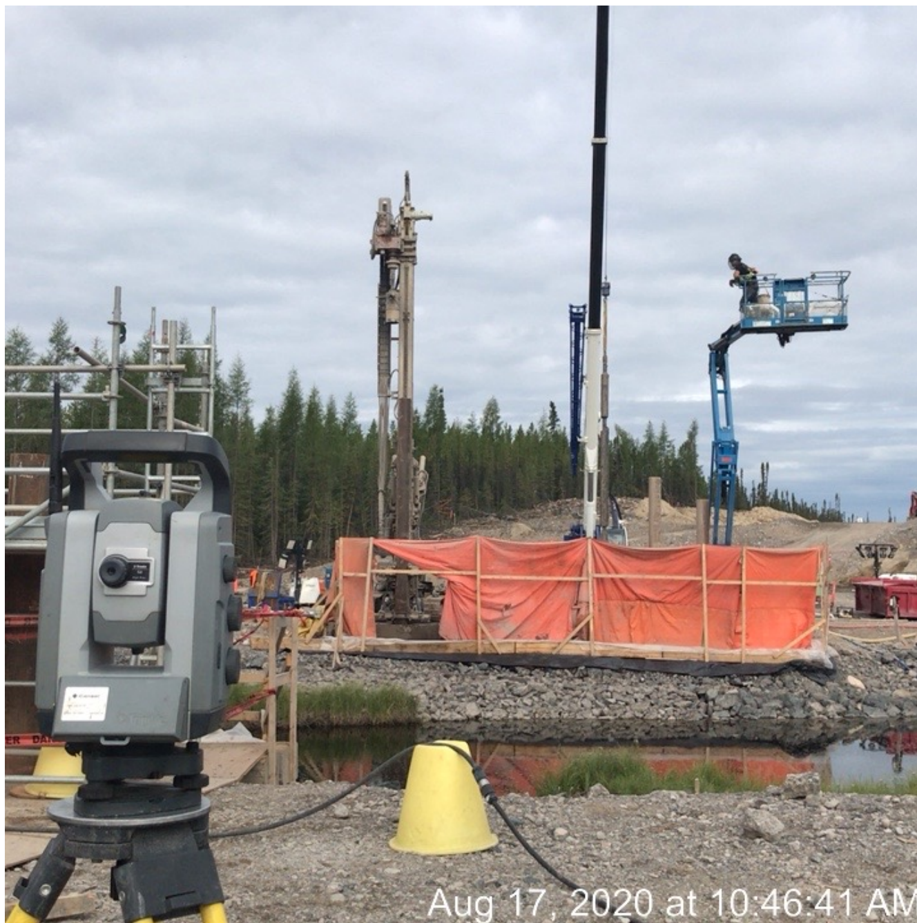
Photo 13. Looking at pile drilling operations and mitigation measures at James River.
