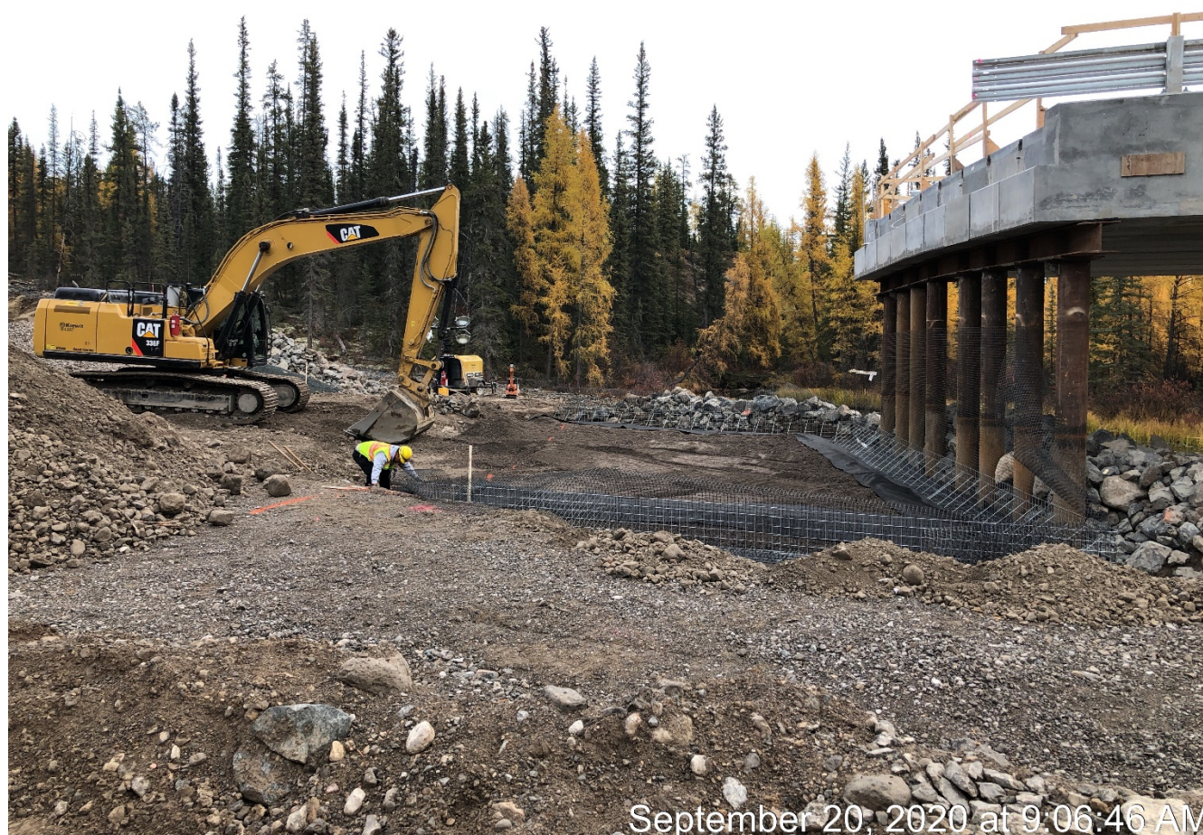
Photo 15. GRS abutment construction on the north side of the James River.
