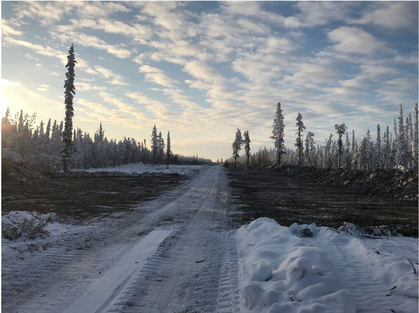
Photo 7. Looking south at stripped section of the TASR from Station 72+540
