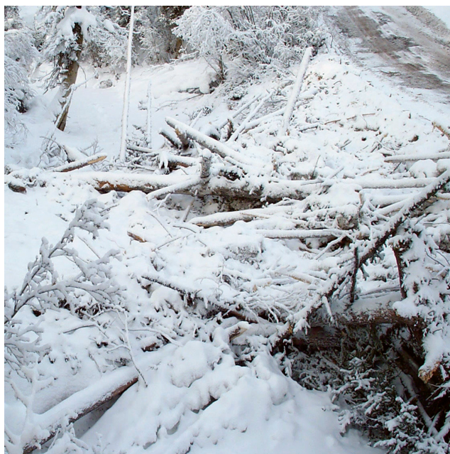
figure 40. A poorly constructed snow fill consisting of mixed brush and snow.
