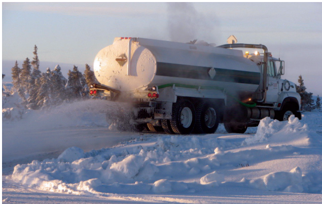
figure 36. The road surface can be built up with ice using a water truck with a sprayer.
