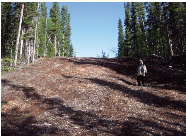
figure 46. Differential settlement can occur in ice-rich permafrost terrain.
