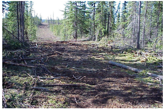
figure 16. Clear only the minimum width necessary for road use.
