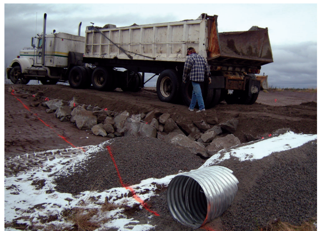
figure 23. This cross drain is covered with coarse-grained granular material for frost protection.
