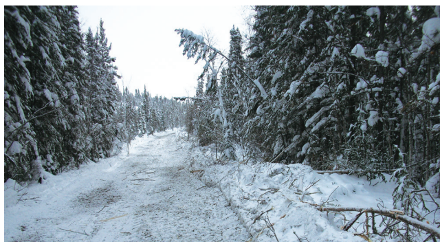
figure 25. Leaners on this recently cleared seismic line should be removed and more snow or ice is required to protect the ground surface.
