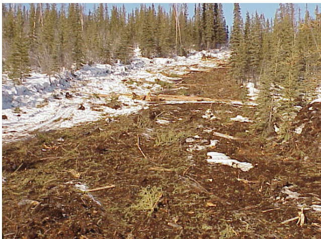
figure 44. Brush can be rolled back across steep slopes to prevent erosion.
