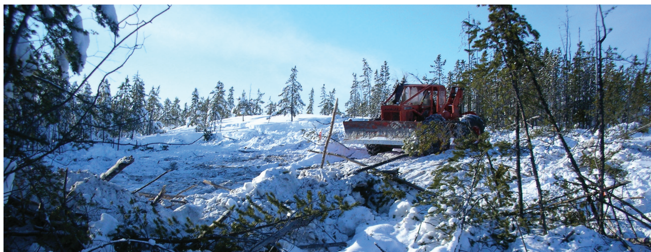
figure 24. Use of a shear blade with a skidder is an acceptable method of clearing in relatively flat terrain.
