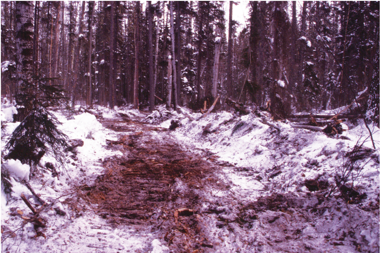
figure 33. On this seismic line, brush is piled in windrows, but standing trees in the piles need to be cut down. More snow or ice is required to protect the ground surface.
