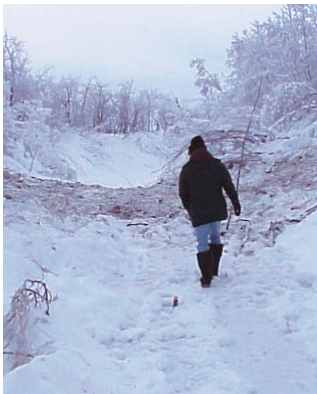
figure 12. Snow fills should be constructed of clean ice or snow, creating a level surface from bank to bank. This snow fill should have been constructed with clean material and more gradual slopes.
