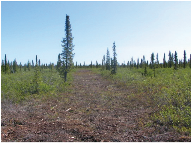
figure 31. A one-year-old seismic line where mulching and scattering was used to dispose of brush.
