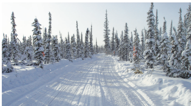
figure 26. An acceptable seismic line with no leaners and adequate packed snow.
