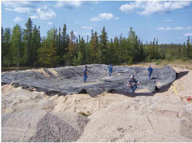
figure 38. A properly lined and bermed area can be used as a secondary containment area for fuel storage.
