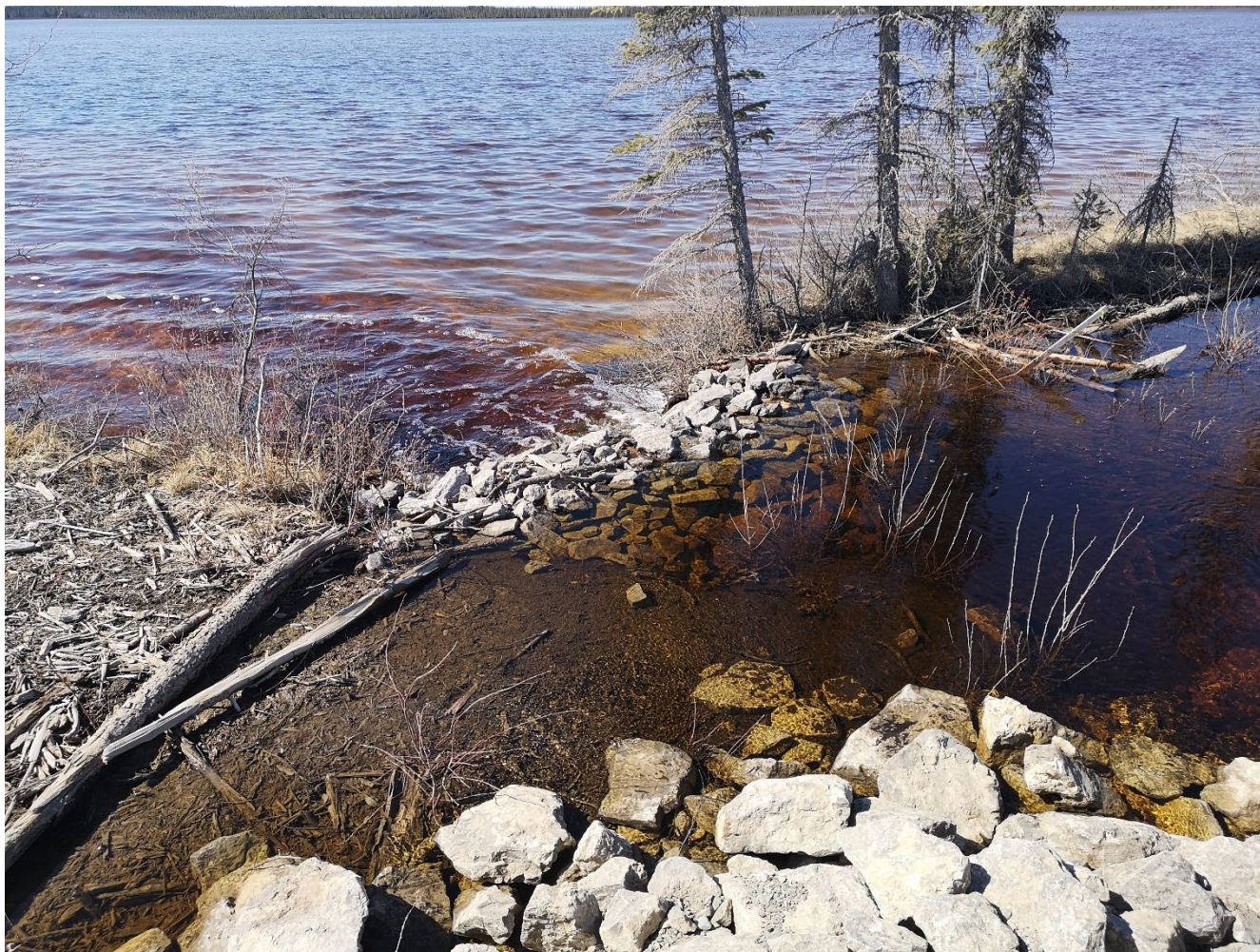
Figure 4-1: Looking at the fish exclusion rock plug installed on the downstream side of the culverts at 46+220
