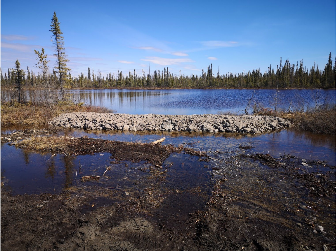
Figure 4-2: Looking at the fish exclusion rock plug installed on the upstream side of the culverts at 46+220
