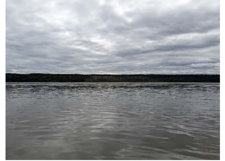
6) Looking at the landslide along the left of the Mackenzie River at PXS-14 (RS 12692).
