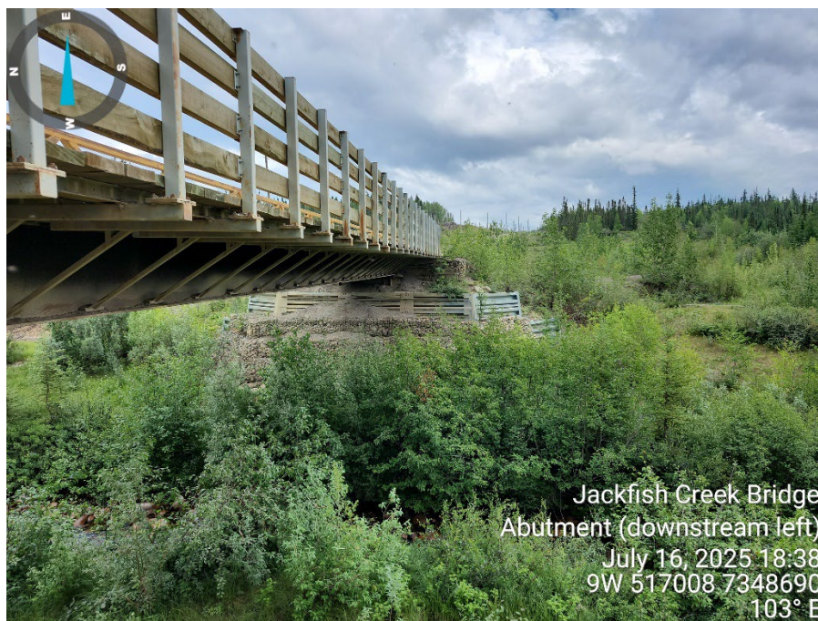
Figure 2: Jackfish Creek Bridge Facing East
