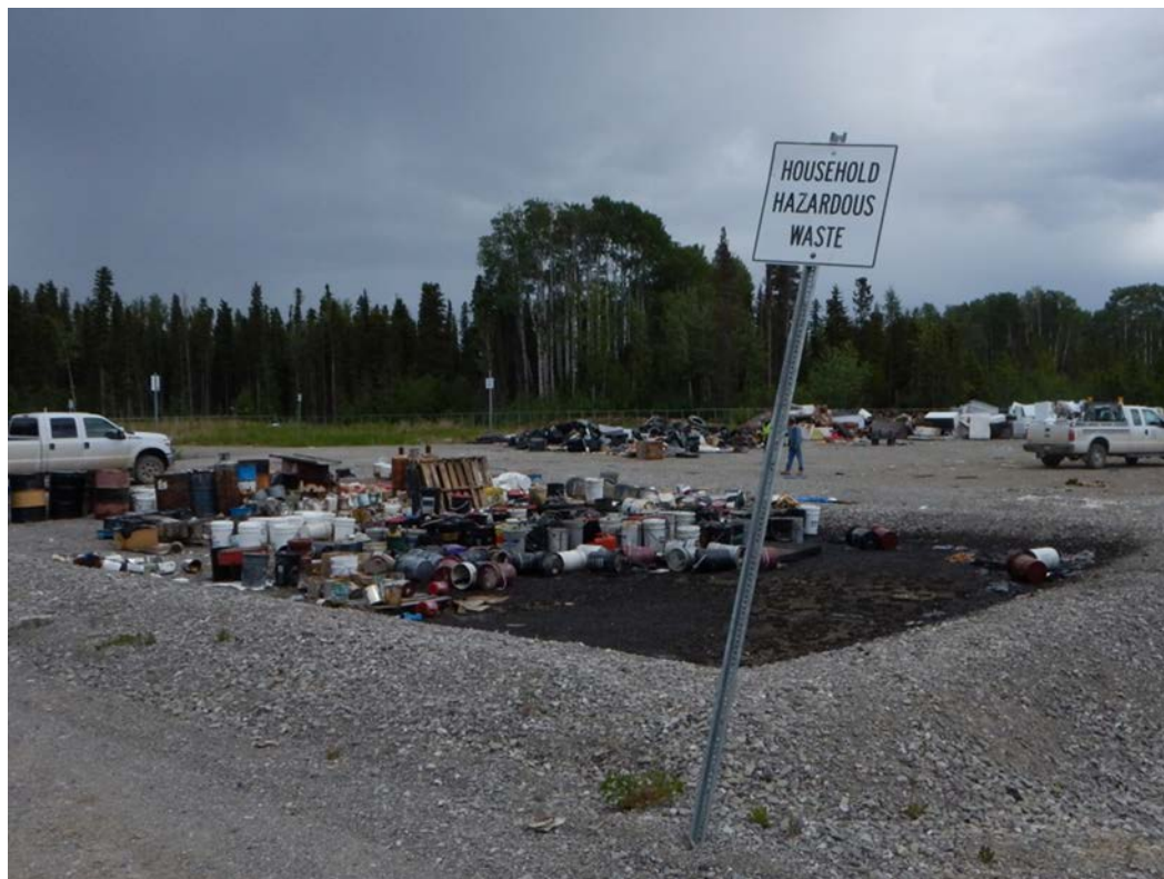
Photo 6: Lined Hazardous Waste Storage Area (Fort Liard)
