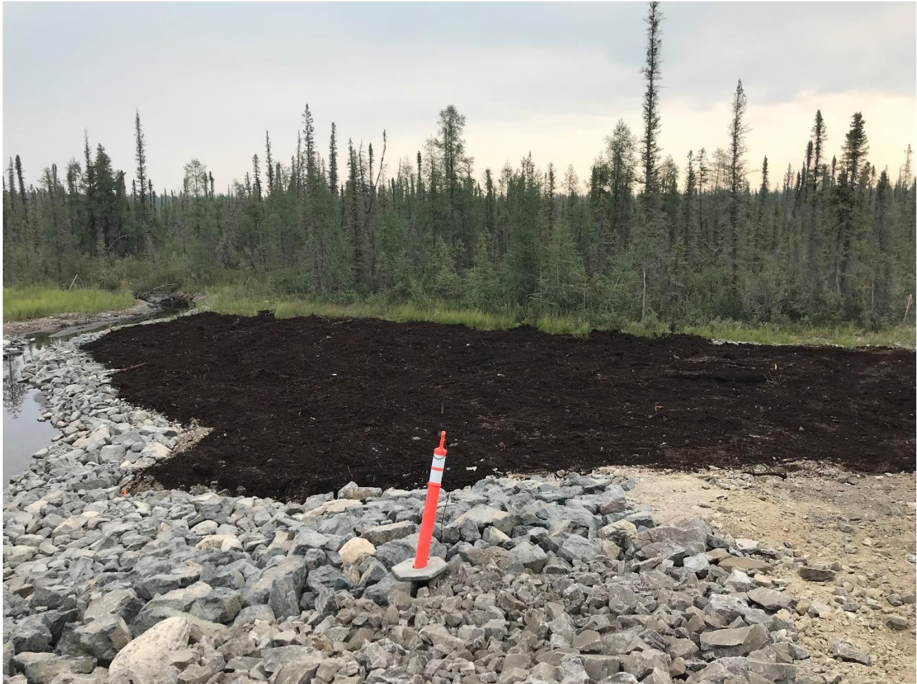
Photo 29. Looking east at the south side of the constructed channel at Culvert 10a after the spreading of organic material
