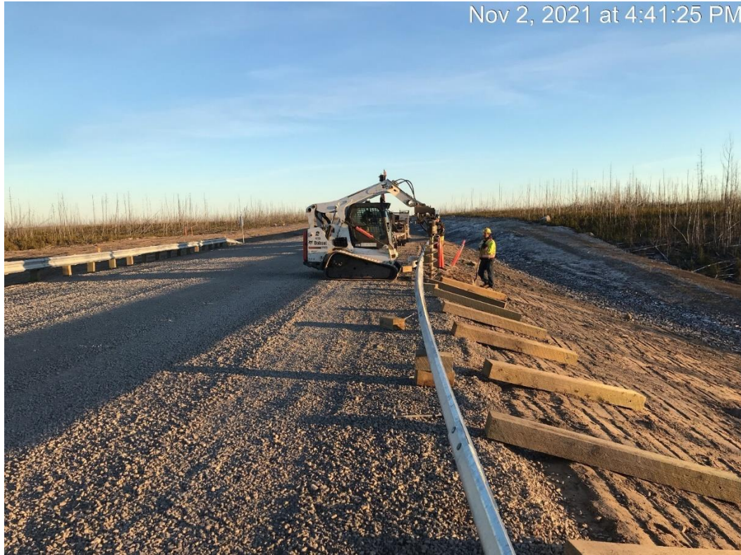
Photo 25. Looking south at the installation of guardrail sections at approximately Station 18+600
