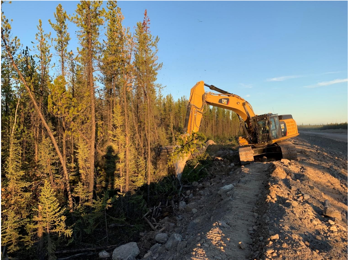
Photo 3. Looking north at clearing along RoW for slope finishing and excess material management at Station 51+300
