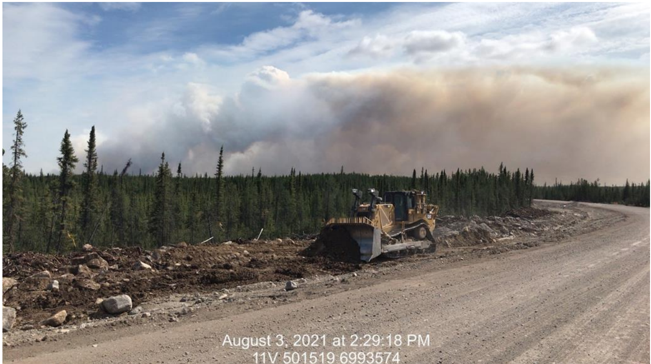
Photo 6. Looking southeast at a dozer shaping ditch line at Station 81+144
