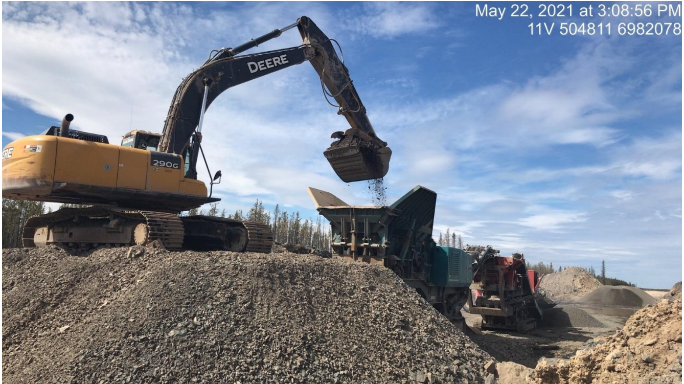
Photo 4. Looking south at the LaPrairie crushing operation at KM 79 road cut - Station 78+383
