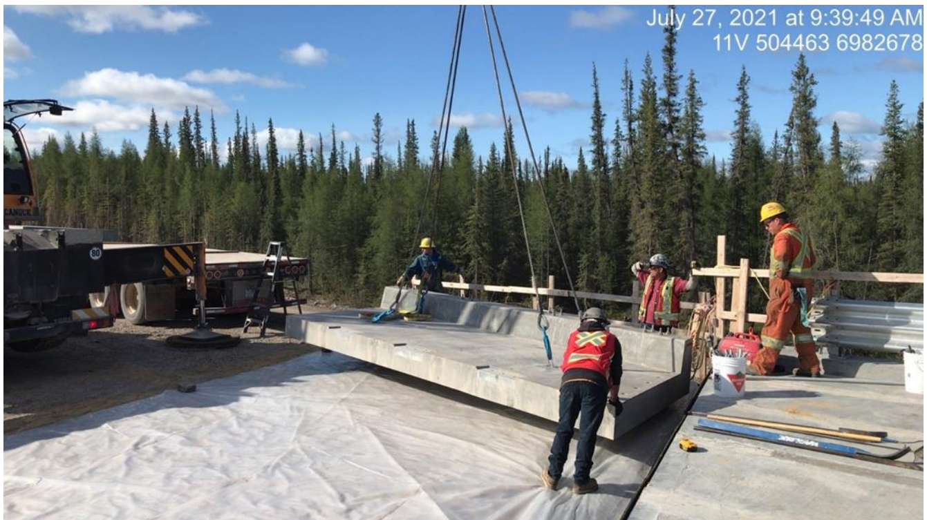
Photo 16. Looking west at the placement of an approach slab at the James River structure
