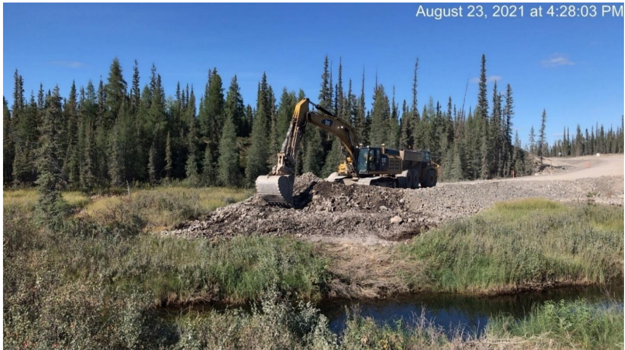
Photo 19. Looking north at the controlled removal of gravel from the temporary access at Duport River
