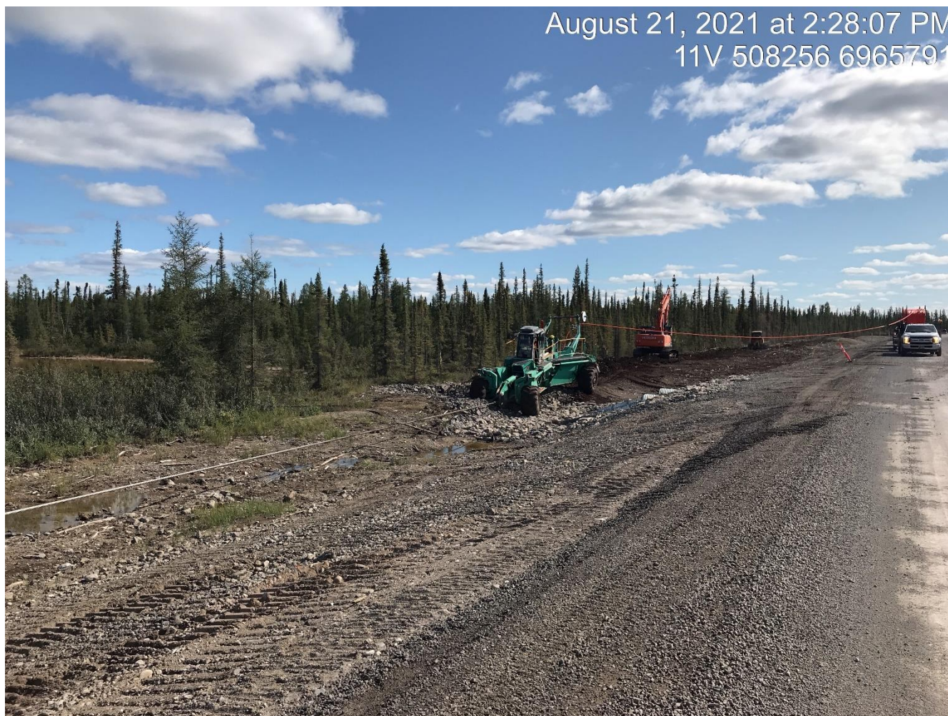
Photo 22. Looking south at conduit plowing around an intermittent watercourse crossing at Station 51+451.
