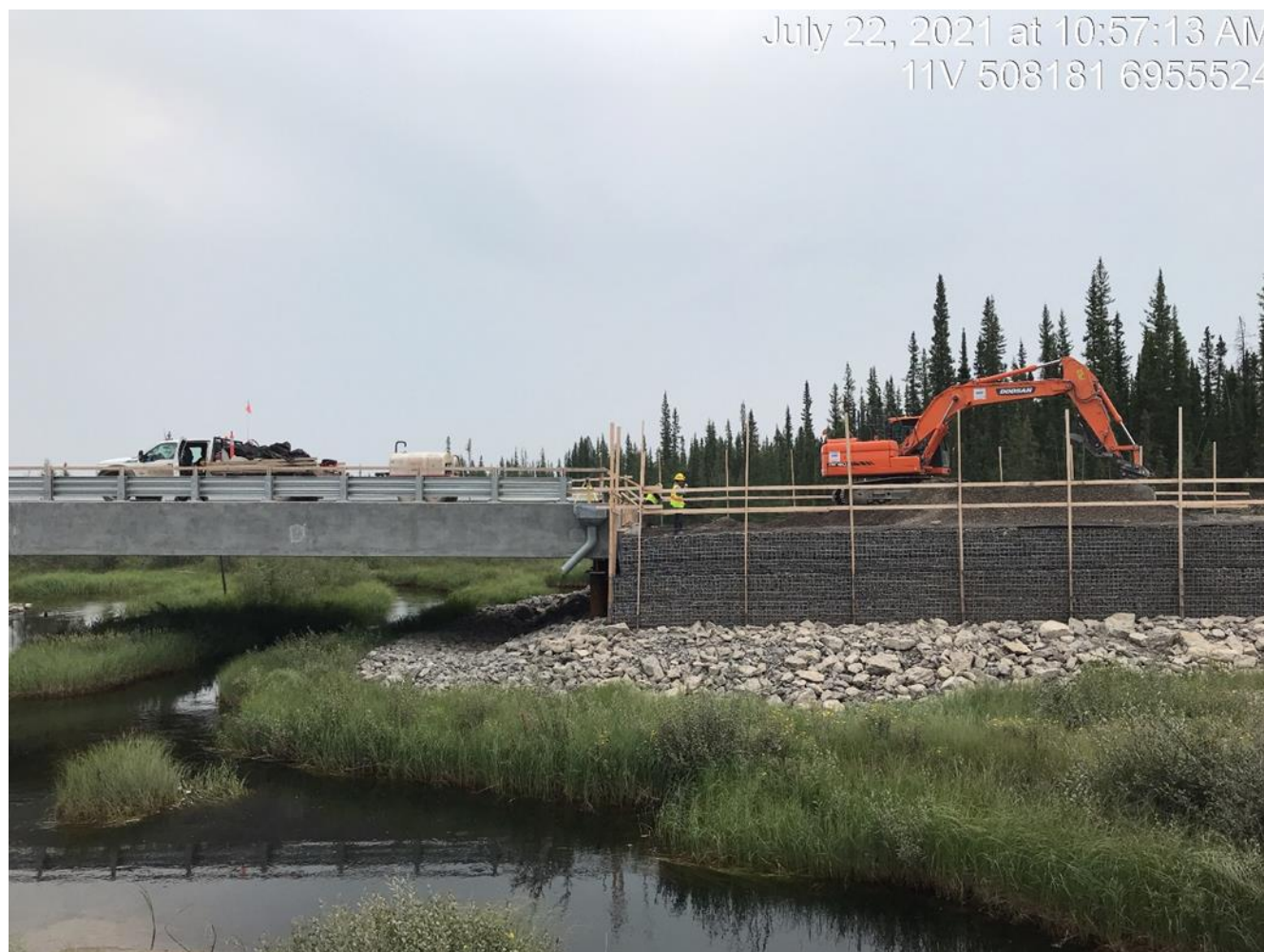
Photo 13. Looking east at the preparation of subgrade prior to the approach slab placement at Duport River (south side)
