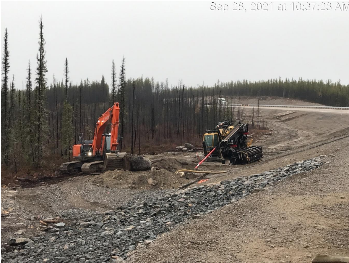
Photo 24. Looking northwest at the directional drilling operation on the north side of the LaMartre River at ~ Station 85+500
