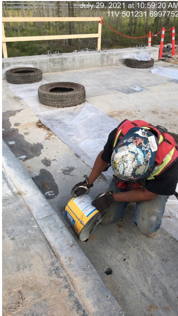
Photo 18. Looking at the pouring of epoxy grout at the approach slab joint with the LaMartre River structure
