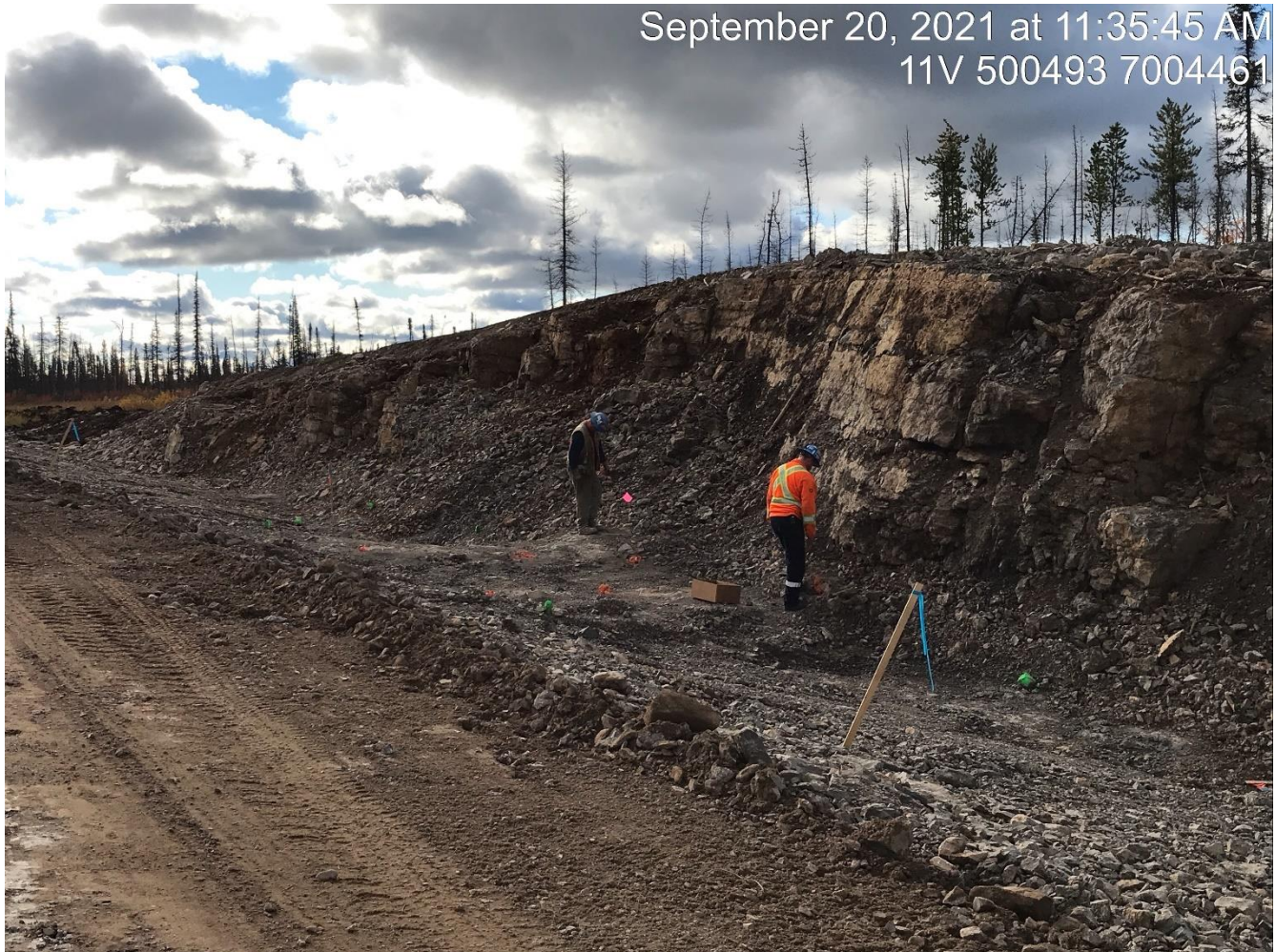
Photo 12. Looking southwest at the loading of holes for a blast at Station 92+634
