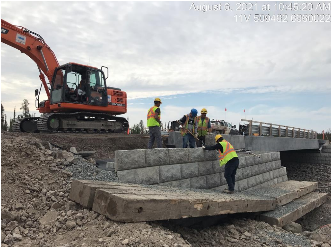
Photo 14. Looking northwest at the completion of the prefabricated concrete facing at the Unnamed River crossing structure.
