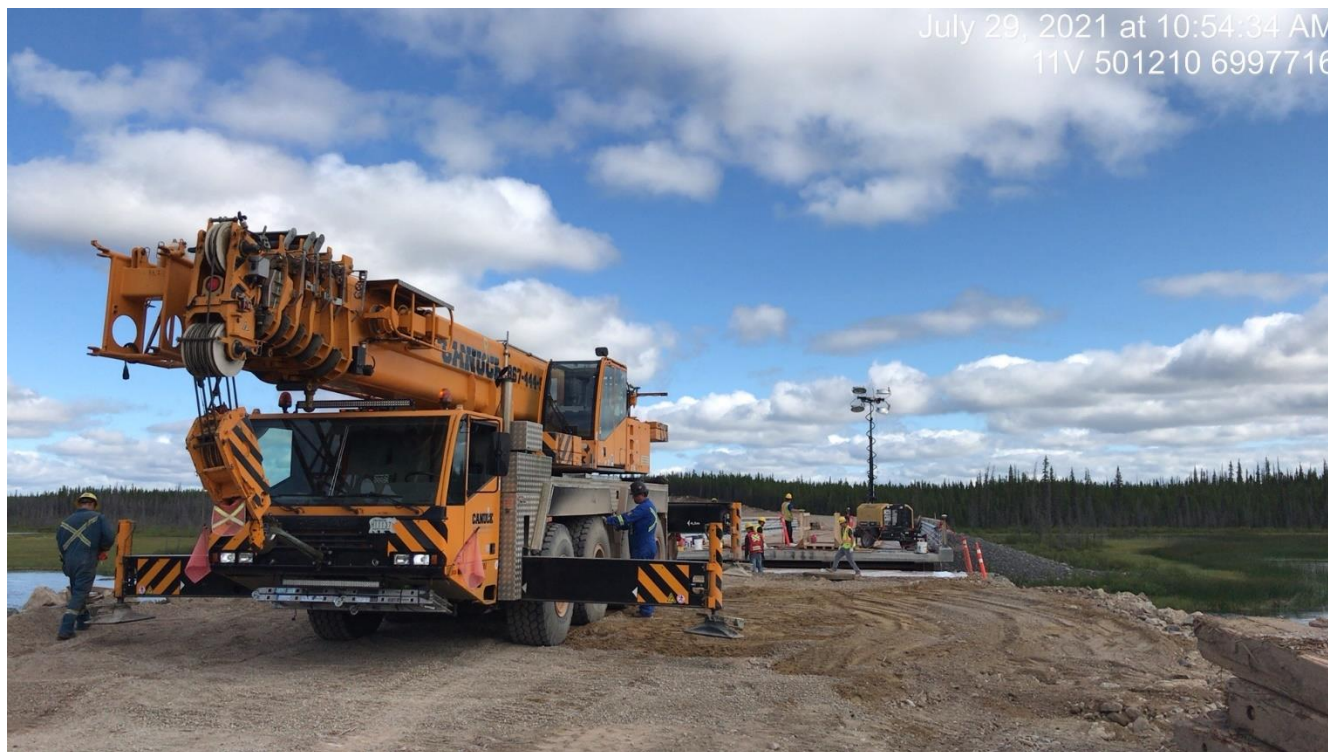
Photo 17. Looking north at the crane set up for the placement of approach slabs on the south side of the LaMartre River
