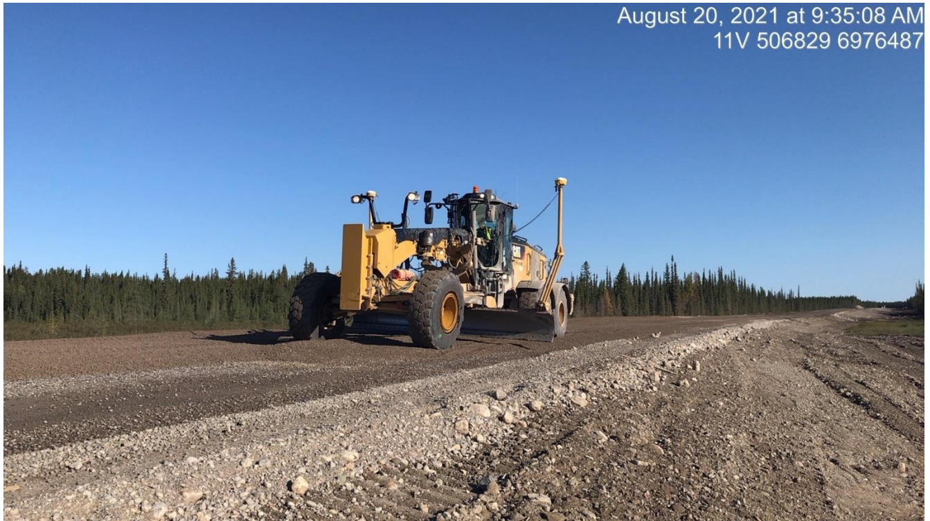
Photo 10. Looking northwest at grader spreading gravel on a section of the TASR at Station 62+683
