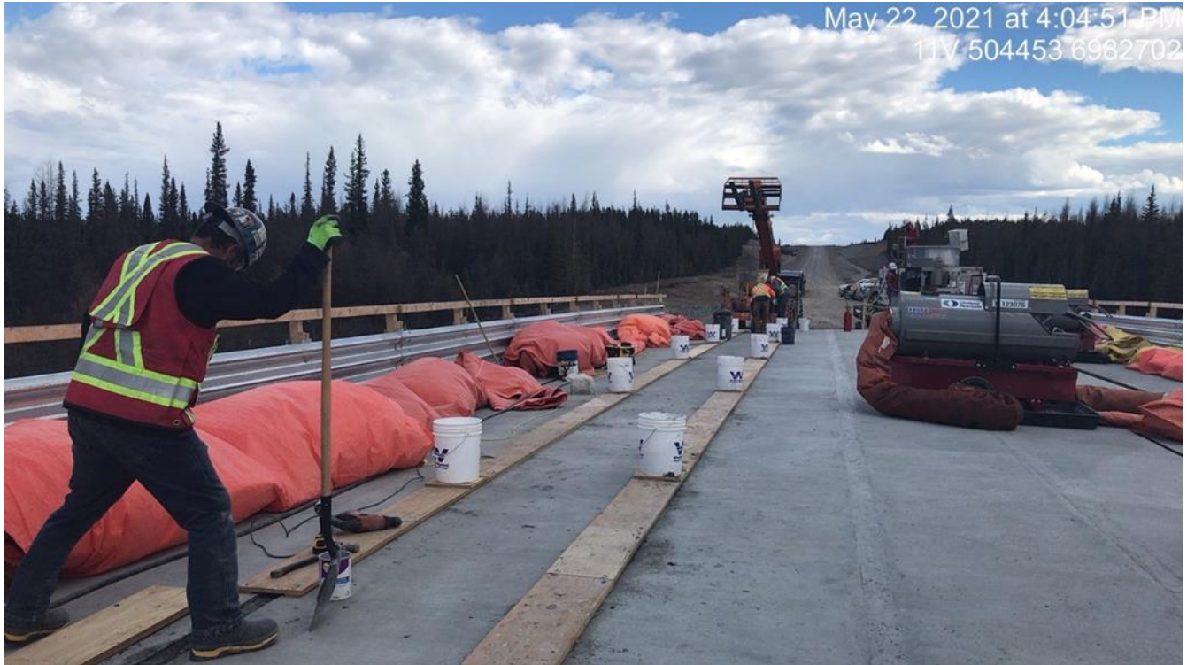
Photo 15. Looking south at grouting of longitudinal deck joints at the James River structure.
