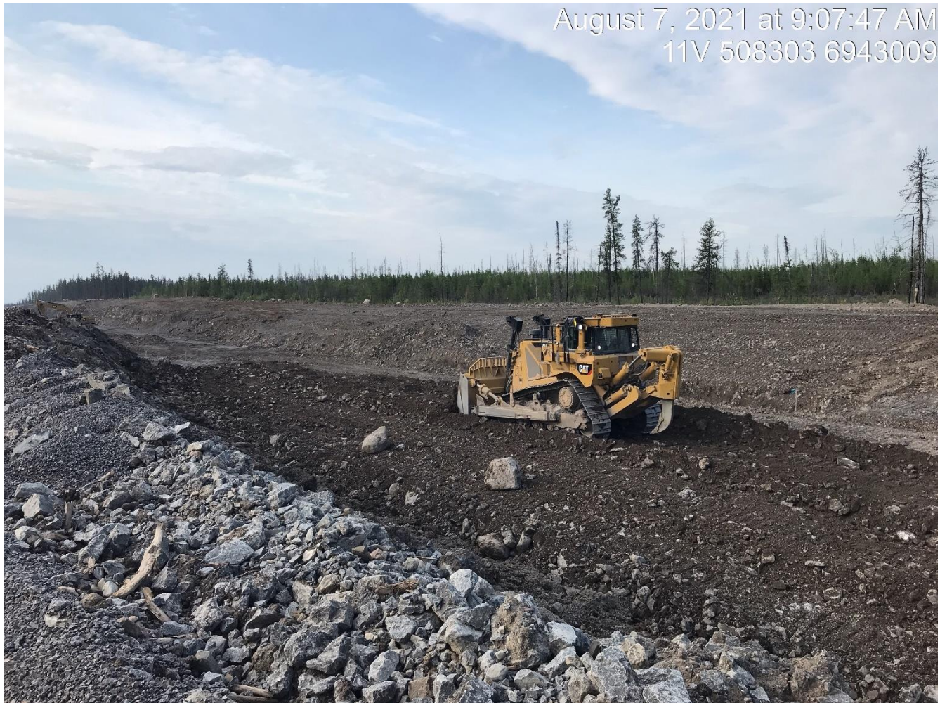
Photo 9. Looking southwest at dozer preparing subgrade through the road cut at Station 35+226
