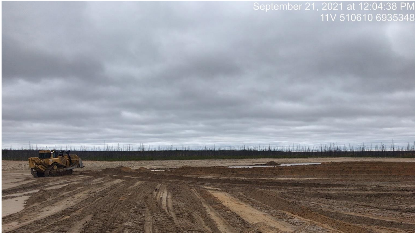
Photo 27. Looking north at dozer doing final grading of the Pit 13C floor
