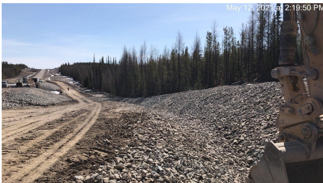
Photo 28. Looking south at the rock lined slopes and west ditch on the north approach of the James River
