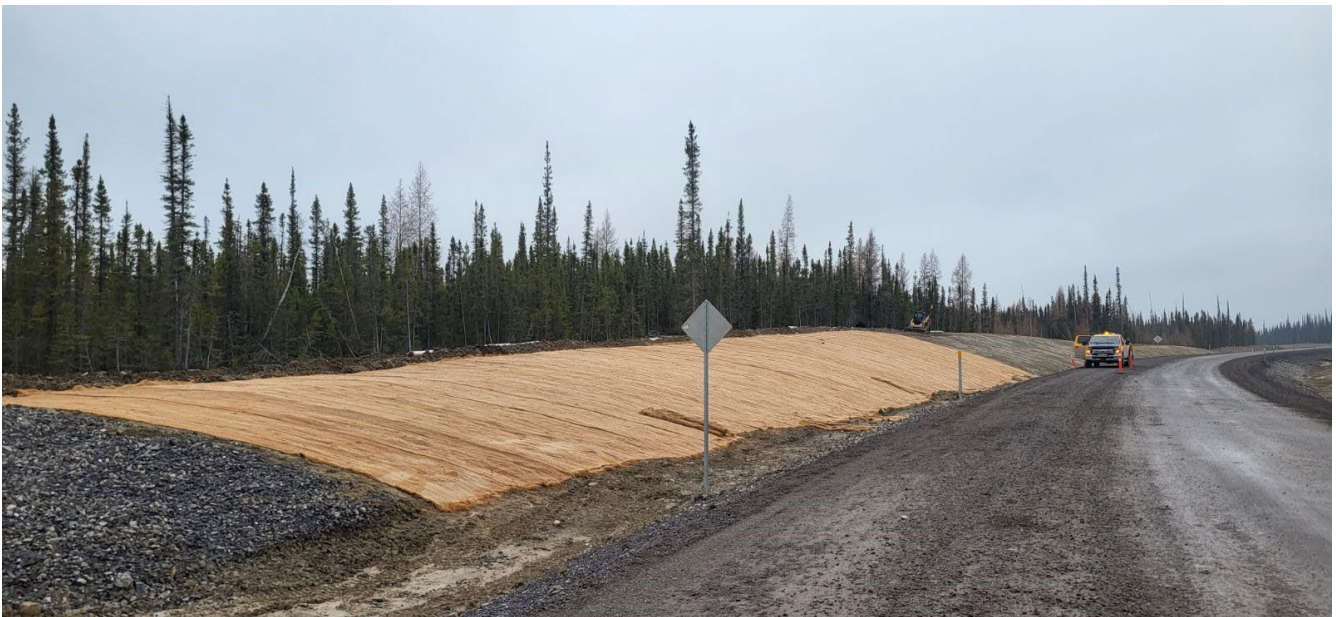
Figure 4-2: Looking south at the progression of erosion control matting installation on the east side south approach.
