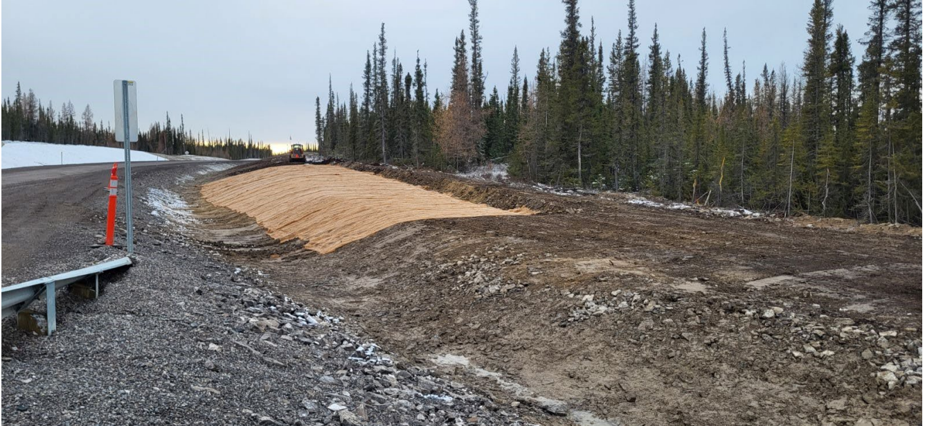
Figure 4-3: Looking south at the progression of erosion control matting installation on the west side, south approach to Duport River.
