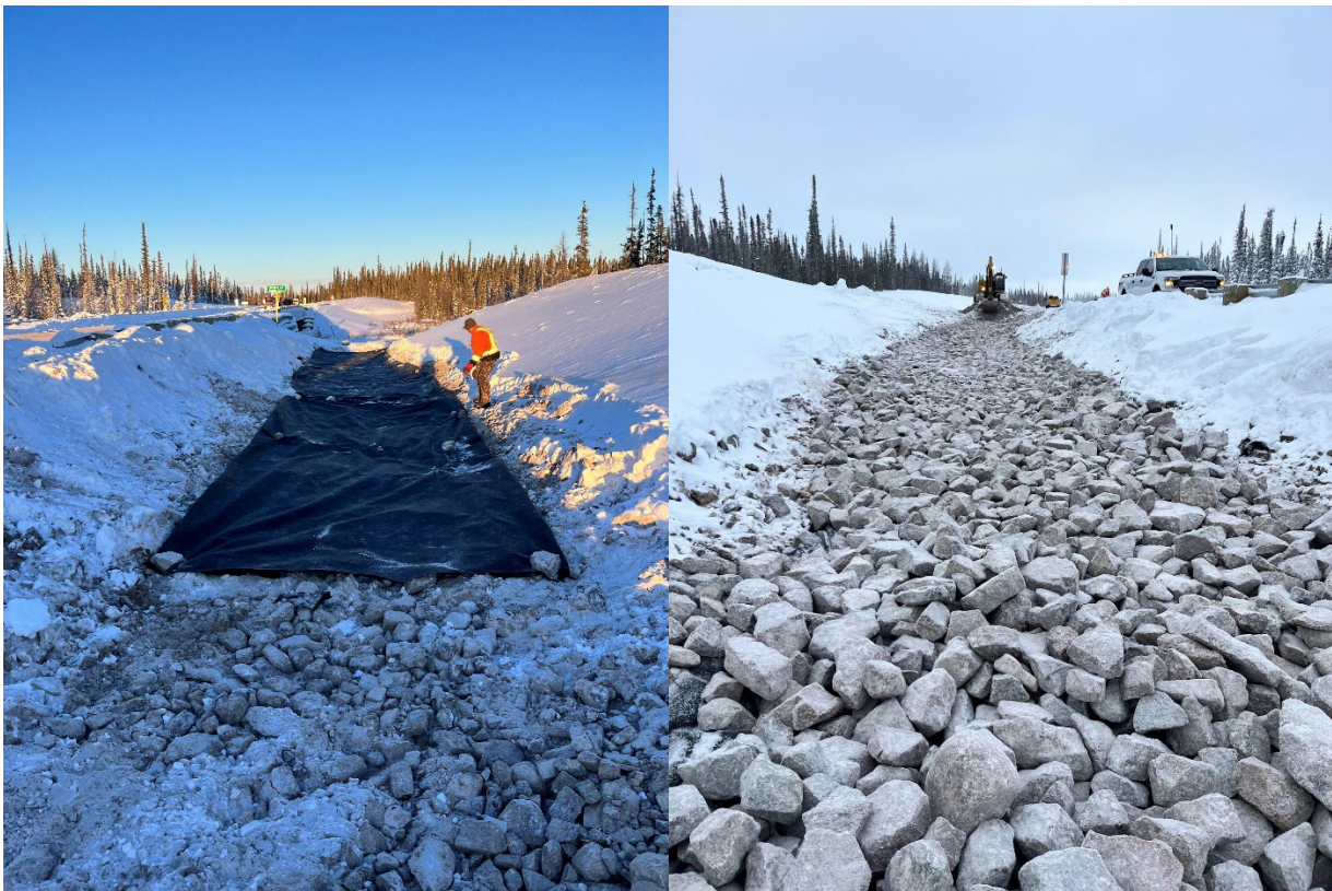
Figure 4-4: Looking north at ditch re-instatement work on the east side, south approach to Duport River.
