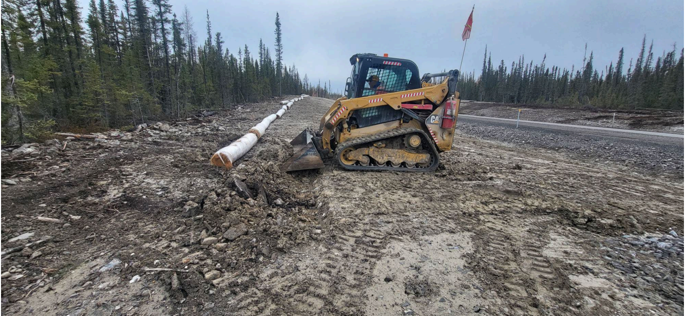
Figure 4-1: Looking south at slope preparation activities for installation of erosion control matting at ~Station 46+220
