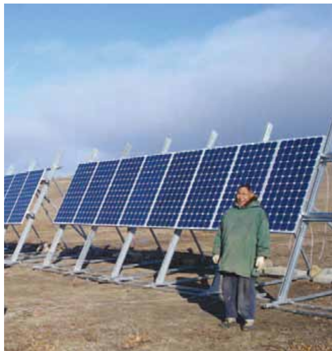
Roger Kuptana, Polar Griz Lodge, Sachs Harbour, 4.3 kW Grid Interconnected, Installed 2010 - Photo Credit: Randall Benson
