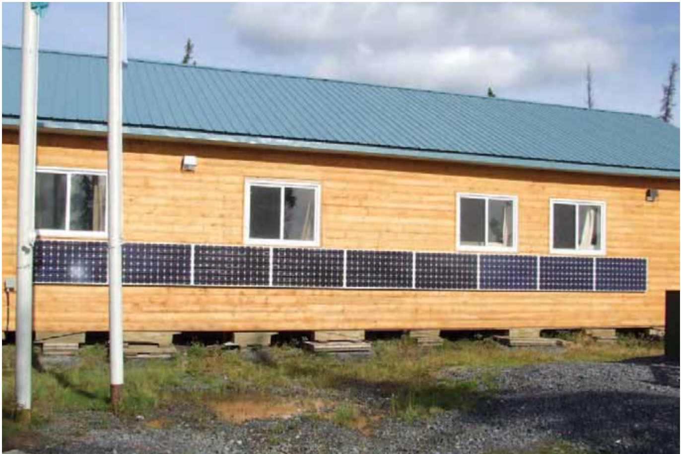
Gwich'in Wellness Camp, 1.7 kW Isolated Diesel Grid Interconnection, Installed 2010 – Photo Credit: Matthew Brost
