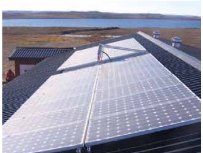
Paulatuk Youth Centre, 5kW Grid Interconnected, Installed 2011 – Photo Credit: Bart Coumont
