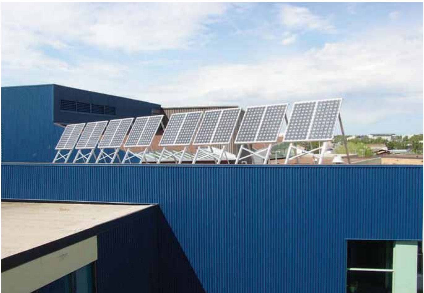
Sir John Franklin High School, 2 kW Grid Interconnected, First Public Grid-tie in the NWT, Installed 2003 – Photo Credit: Wade Carpenter
