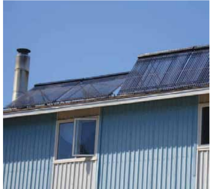
Solar Hot Water Heating – Photo Credit: Tom Gross
