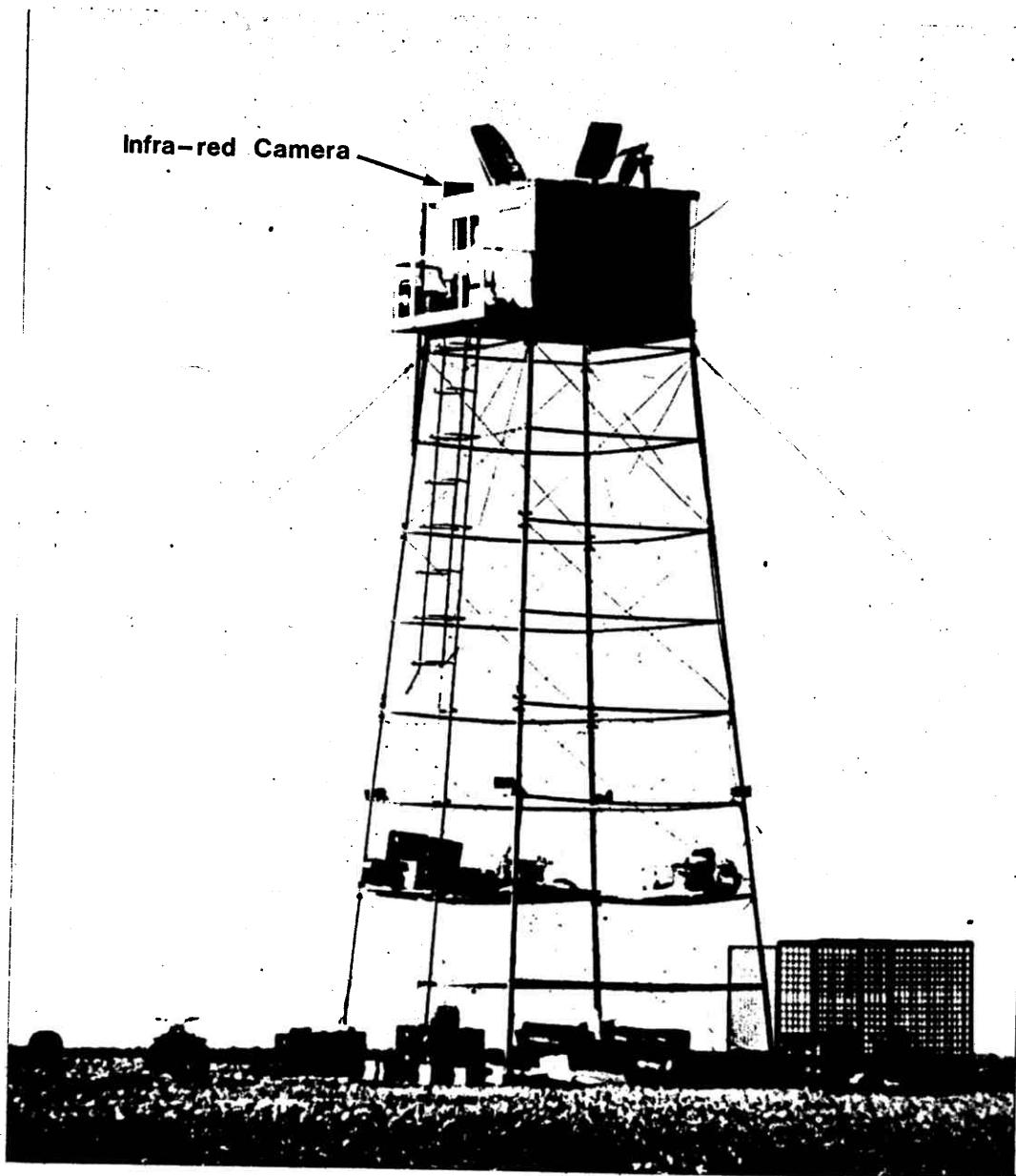
Figure 2. Observation tower/living quarters with infra-red detection unit mounted roof, Cape Churchill, Manitoba, 1984.
