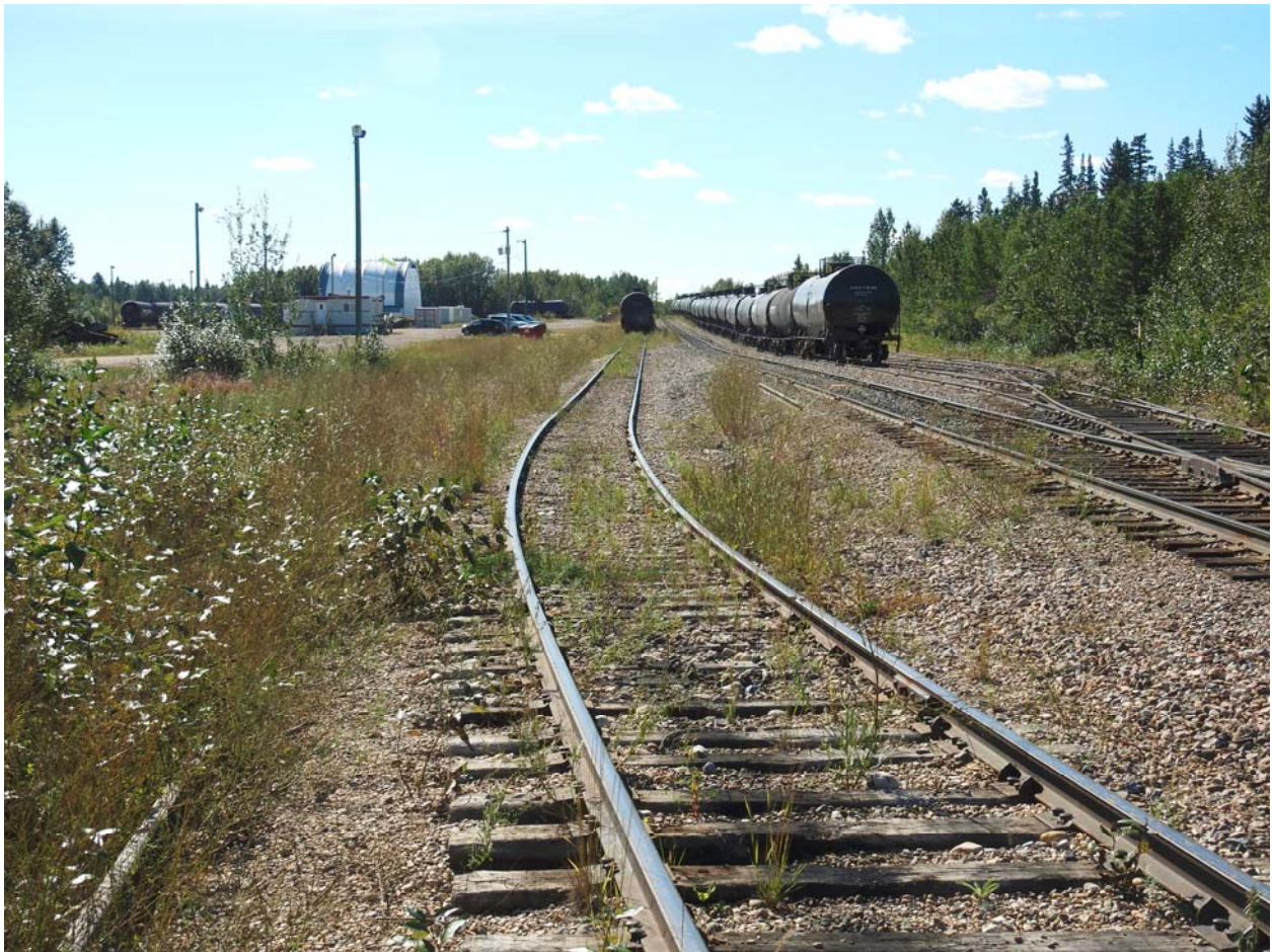
Figure 8. Railway survey site at Hay River.
