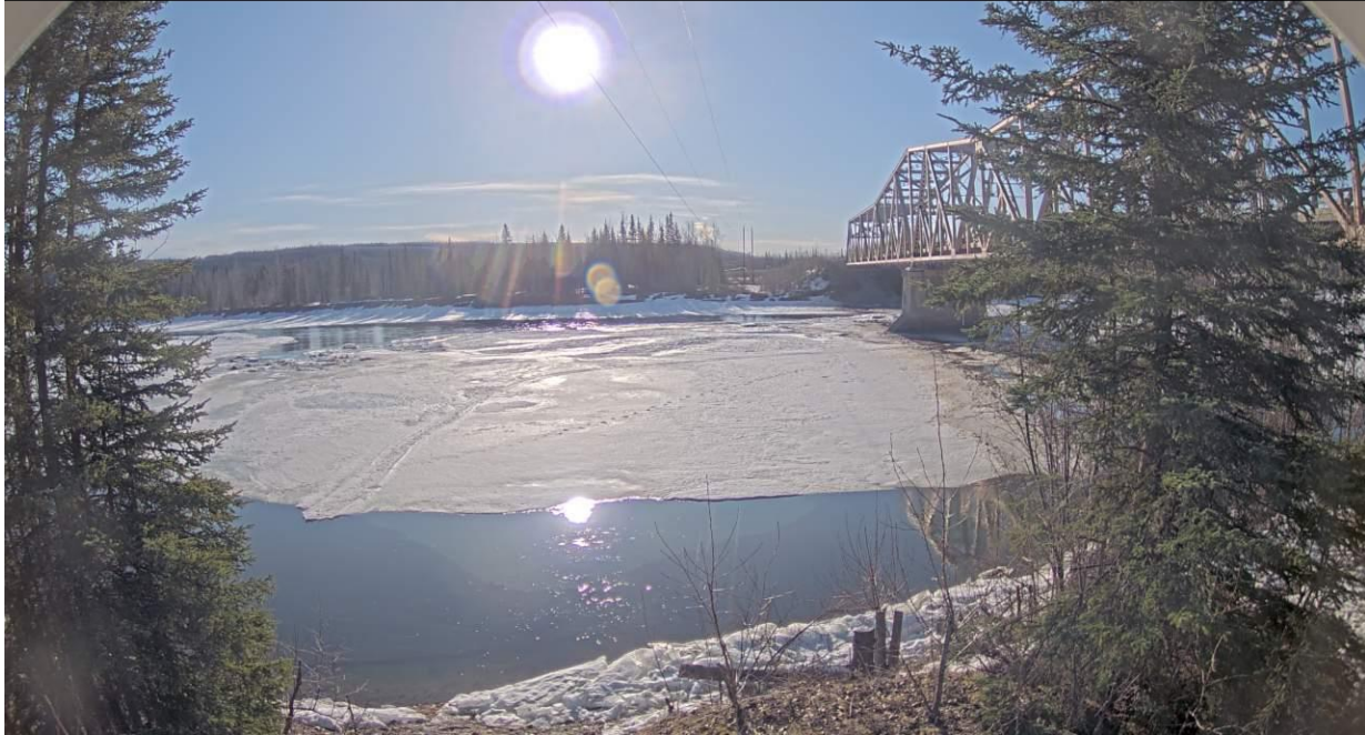
Above - Liard River at Upper Crossing [10AA001] hydrometric gauge photo from May 1 at 08:02. Photo courtesy of Water Survey of Canada and Government of Yukon.
