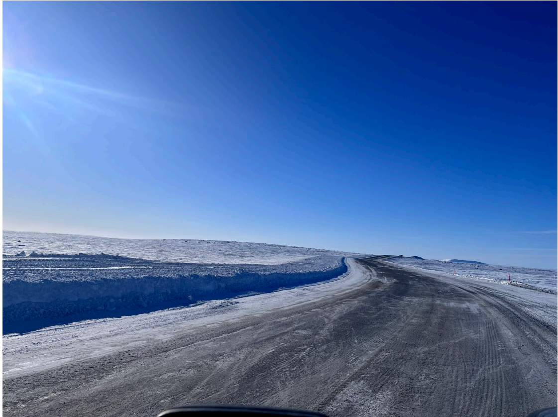
Image 2: Example of a leveled snow berm along the haul road less than 1 meter in height.
