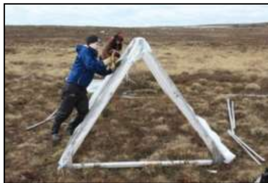
Photo 5: Building greenhouses in Research Valley.
