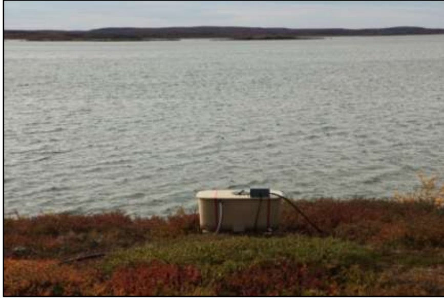
Photo 7: New greywater holding tank.
