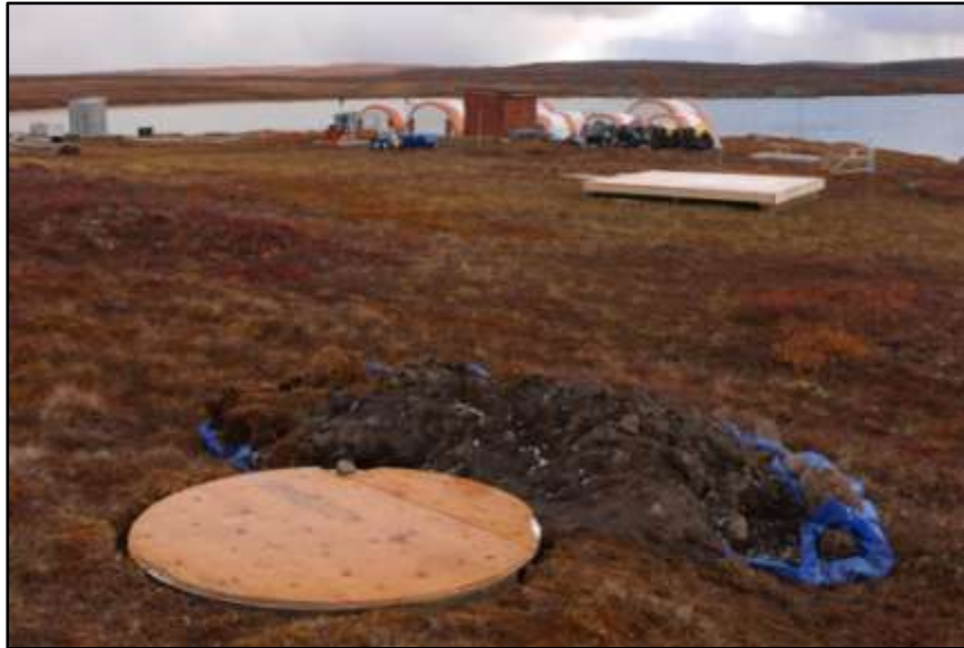
Photo 8: New, covered greywater pit.
