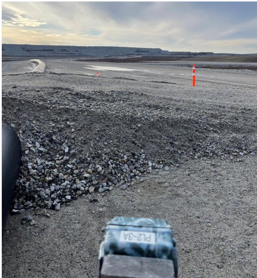
Figure 4: Caribou crossing ramp over the Point Lake Stage Two Dewatering Pipeline on the Lac du Sauvage Road at the Ekati Diamond Mine, June 2023. Note wildlife monitoring camera 3A mounted on a wooden post in the foreground. Misery Waste Rock Storage in the background.
