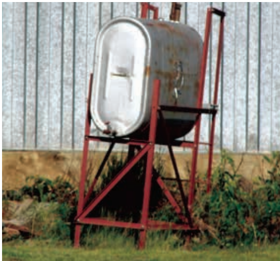
A wobbly or leaning tank can cause a break in your fuel line
