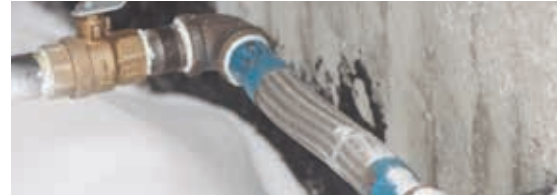
Flex hose helps prevent broken fuel lines
