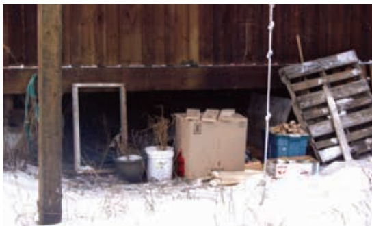
Storing materials under your house can encourage permafrost thaw
