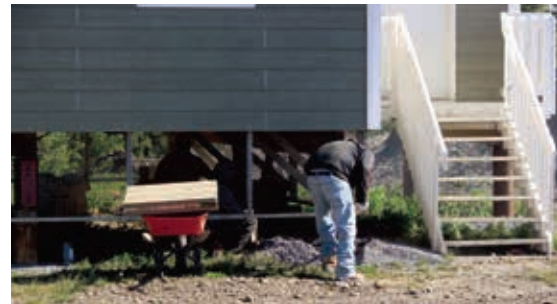
Gravel pad should be domed to shed water
